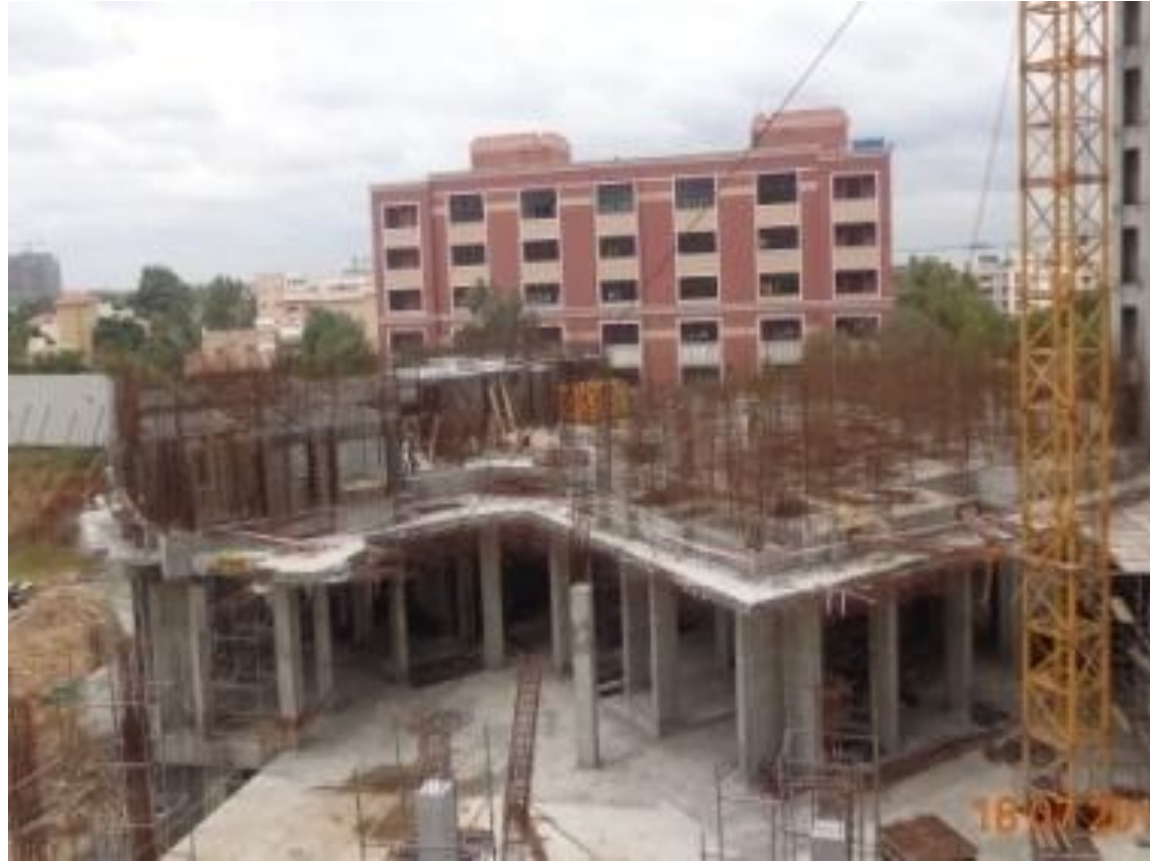
TOWER G : Level 1 in Advanced Stages of Progress.
