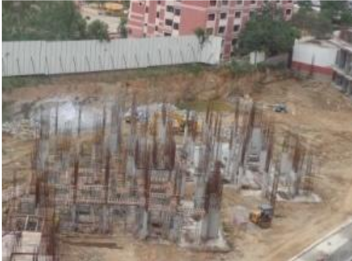
TOWER H : Lower Basement Works in Progress.
