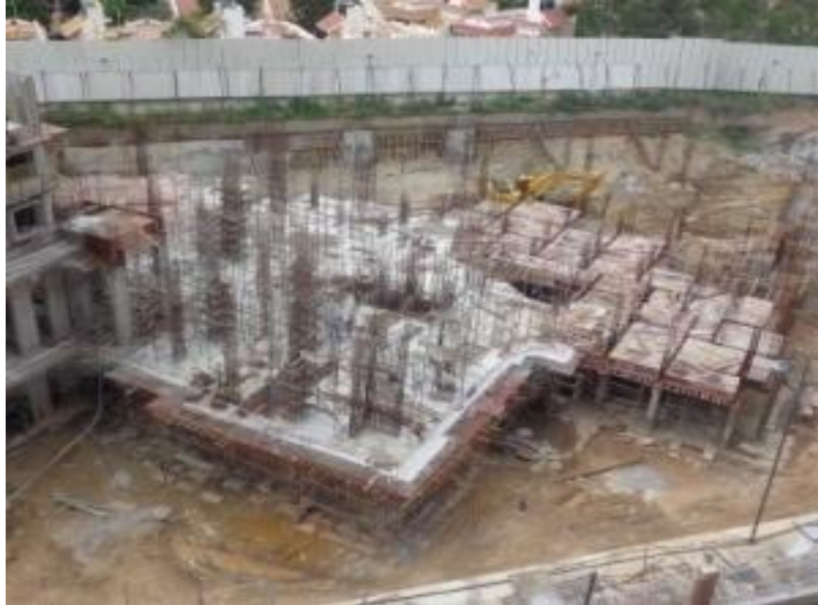
TOWER J : Lower Basement in Advanced Stages of Progress.
