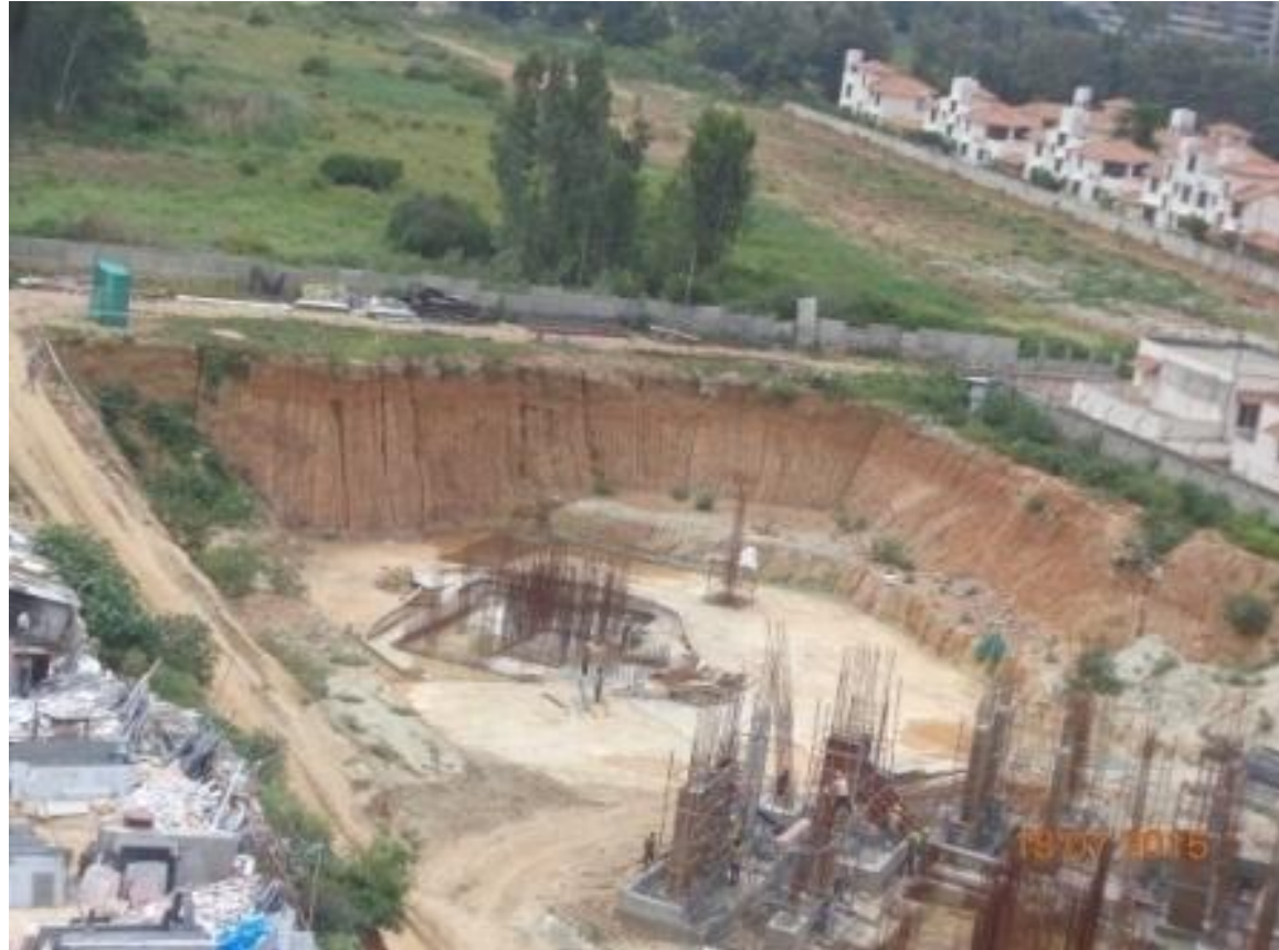
TOWER N : Foundation Works in Progress
